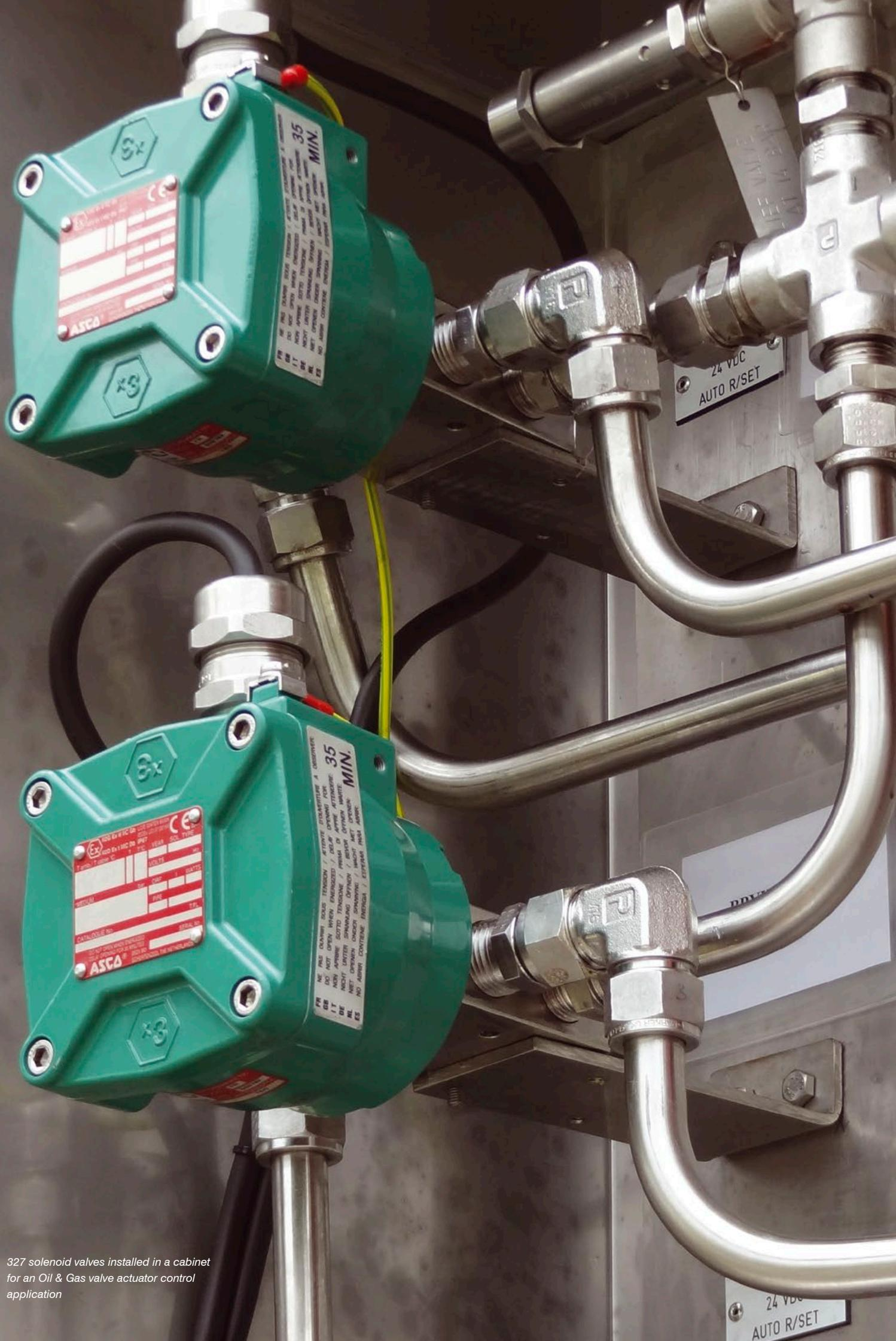
327 solenoid valves installed in a cabinet for an Oil & Gas valve actuator control application
