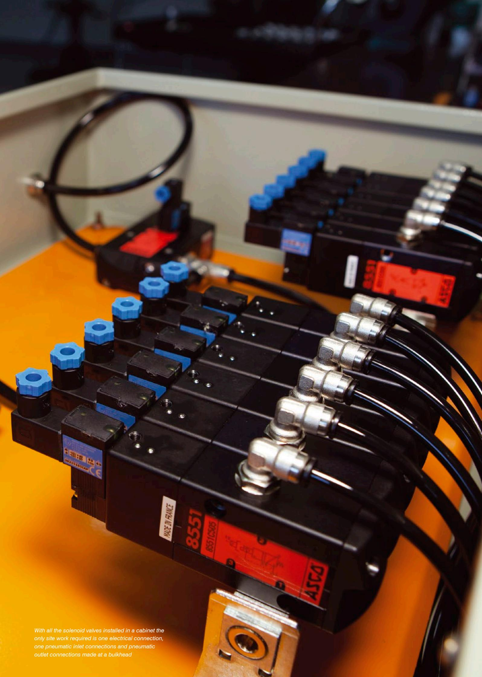
*With all the solenoid valves installed in a cabinet the only site work required is one electrical connection, one pneumatic inlet connections and pneumatic outlet connections made at a bulkhead*
