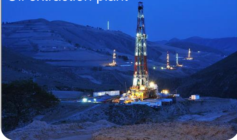
Oil extraction plant
