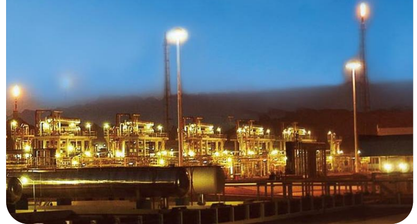
Oil & Gas refineries plant
